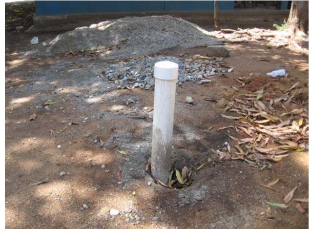
Completed borehole waiting for pump
